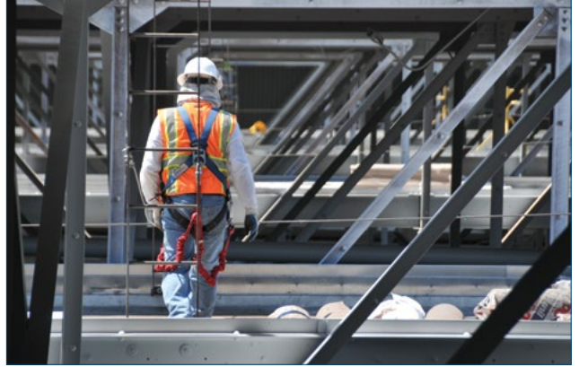
Technician properly tied off while working at California Steel Industries in Fontana, Calif., USA.
